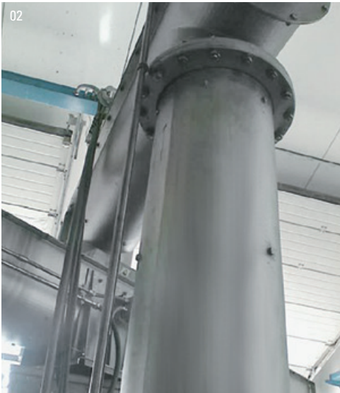
01 _ Screenings conveyance 02 _ Vertical conveyor detail (transition to horizontal) 03 _ Sludge conveyor system
